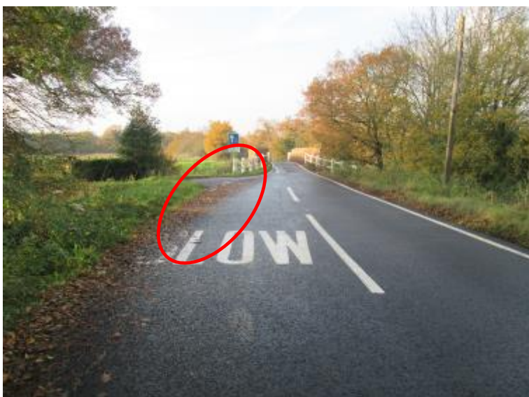
Image 1 – Northbound approach to bridge (road narrows on nearside; also see detriutus on nearside)
