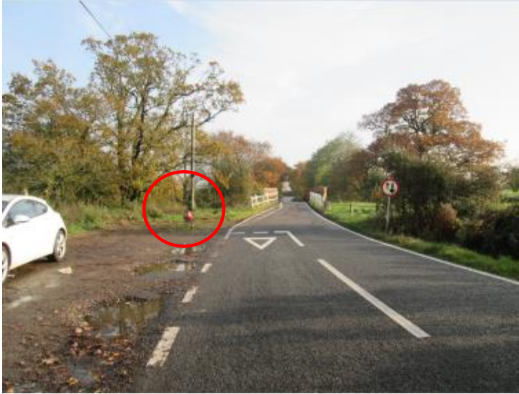
Image 3 – Southbound approach to bridge (road narrows from nearside only and damaged sign)
