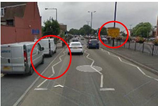
Image 5 – South-eastbound approach (parked vehicles masking pedestrians approaching the crossing and temporary diversion route sign on central reserve)
